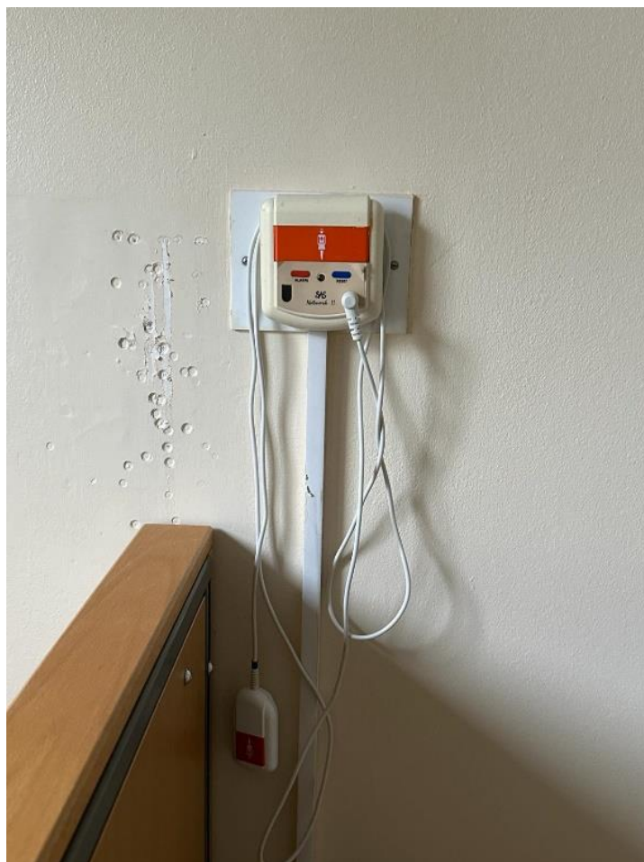
Figure 4: Emergency alarm observed in bedrooms located next to the bed.
